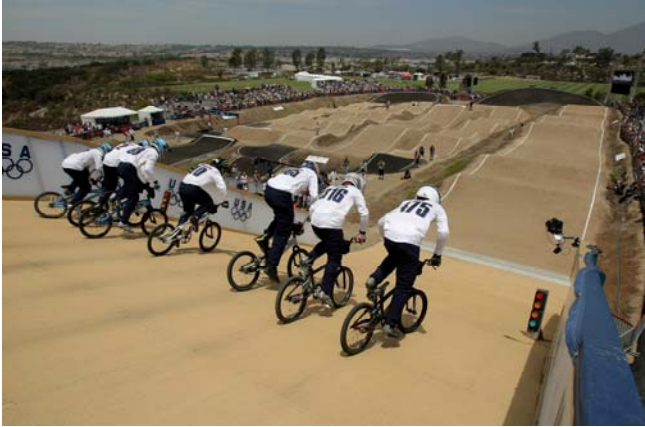
UCI Olympic start tower (9 meters/26 foot height) with eight rider Pro Gate starting system. Overall track length is 370 meters for the women and 390 meters for the men.
